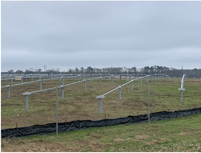
Fig. 1. Nevados trackers being installed on a hill. Angle changes occur along the torque-tube axis at each pile location which allow the Tracker to follow the terrain underneath without the need to level the site.
